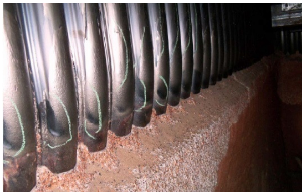
Fig 1 Shows erosion observe on kick off zone
